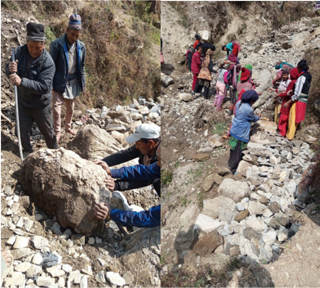
Community members volunteered to construct a walking trail in Gaumul rural municipality, Bajura
