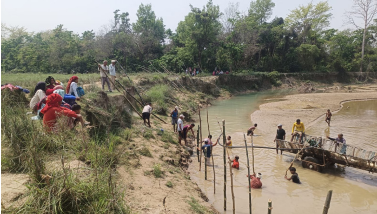
Tole members took an initiative to construct bio-embankment using local resources i.e., bamboo and sand racks at Jaljaliya, Bhajani rural municipality, Tikapur
