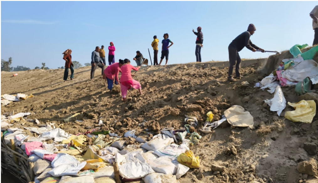
Tole members took an initiative to construct bio-embankment using local resources i.e., bamboo and sand racks at Jaljaliya, Bhajani rural municipality, Tikapur
